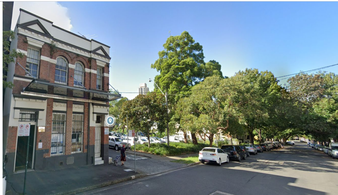
Facing south along Cope Street Left: Wyanga 35 Cope St - Wyanga Aboriginal Aged Care Inc
